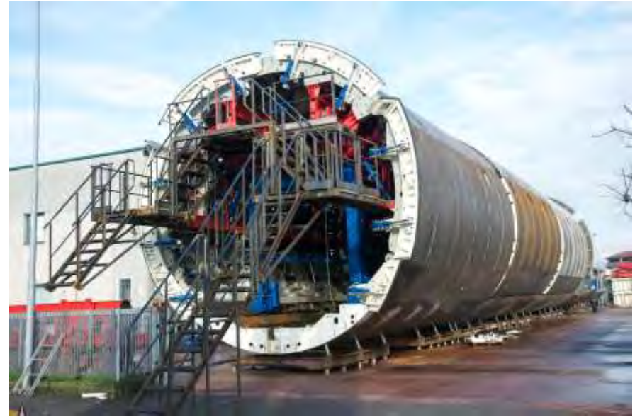
Secondary Lining Shutters Under Construction
