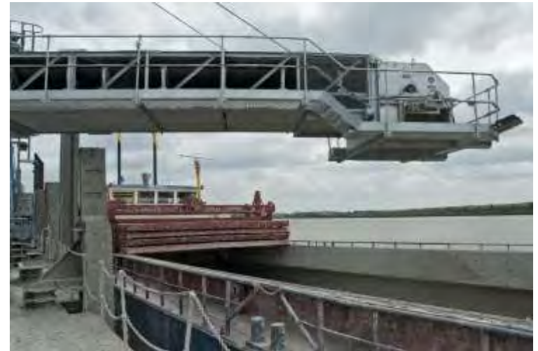
Barge Operations at Beckton Jetty
