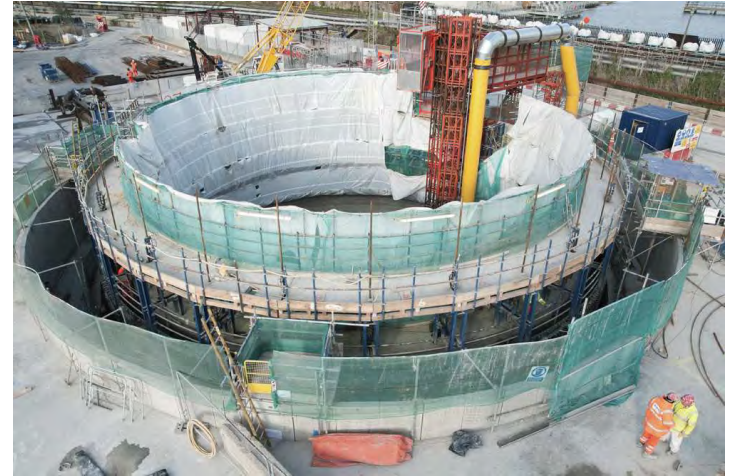
Slipform rig reaching top of Overflow Shaft
